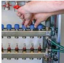
6. Once finished, close the valve and open the next valve at the same time.
