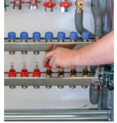
4. Remove the seal caps and open all flow meters.
