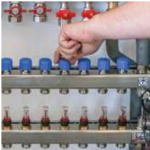
5. Open the valve for the circuit to be flushed and close all other valves. Turn on the water supply.
