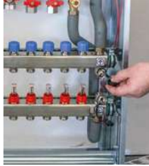
2. Gently open the fill and drain valves.
