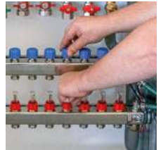
8. Open all valves and flow meters. Install the sealing caps and open the ball valves.
