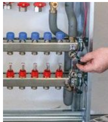
2. Gently open the fill and drain valves.
