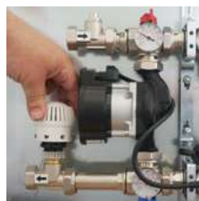
8. Set the thermostat to the desired temperature. (see thermostat scale p. 2)
