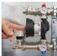
5. Set the pump to differential pressure constant and the desired delivery head.
