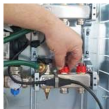
8. Open all valves and flow meters. Install sealing caps and open the ball valves.
