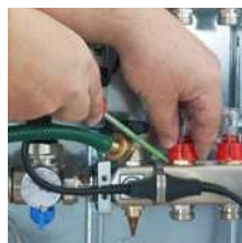
4. Remove the sealing caps and open all flow meters.
