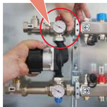
1. Mount the screw connection parts and control unit to the manifold using the enclosed seals.
