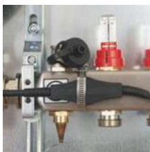
7. Mount STB-A on the supply manifold bar.
