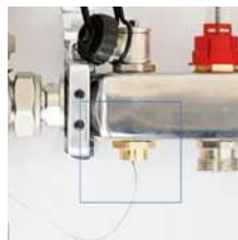
4. Mount the remote sensor with immersion sleeve or hose clamp to the supply manifold.
