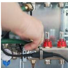
2. Open the filling and drain valves slightly.
