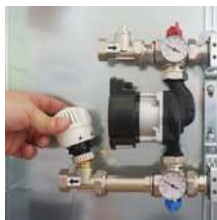
3. Mount the thermostatic head on the control valve in the return pipe.
