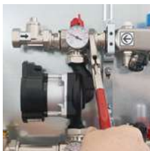
2. Tighten both screw connections.
