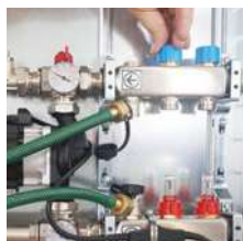
5. Open the circle to be flushed and close all other circles. Turn on the water supply.
