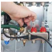
7. Turn off the water supply. Close the fill and drain valves. Remove the hoses and put the caps on.
