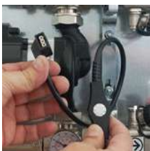
6. Connect the pump with STB-A to the power supply.
