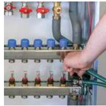
7. Stop the water supply. Close the fill and drain valves. Remove the hoses and replace the caps.
