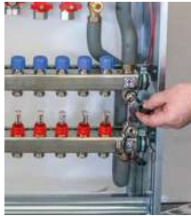
2. Gently open the fill and drain valves.
