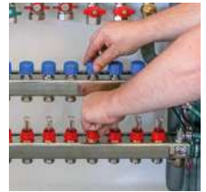
8. Open all valves and flow meters. Install the sealing caps and open the ball valves.
