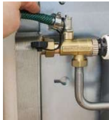
2. Gently open the fill and drain valves.
